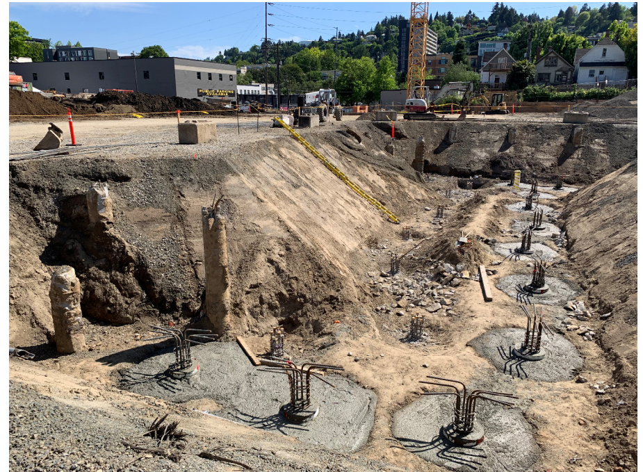
Orchestra Pit Excavation
