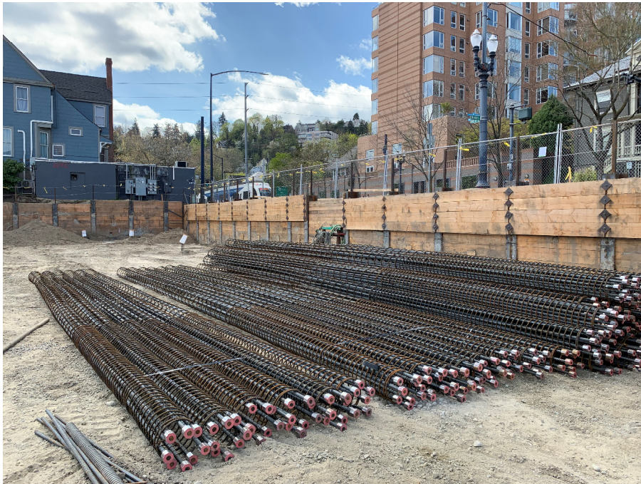
Rebar Cages for Deep Pilings
